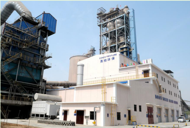
Industrial solid waste disposal project in Fuping, Shaanxi
