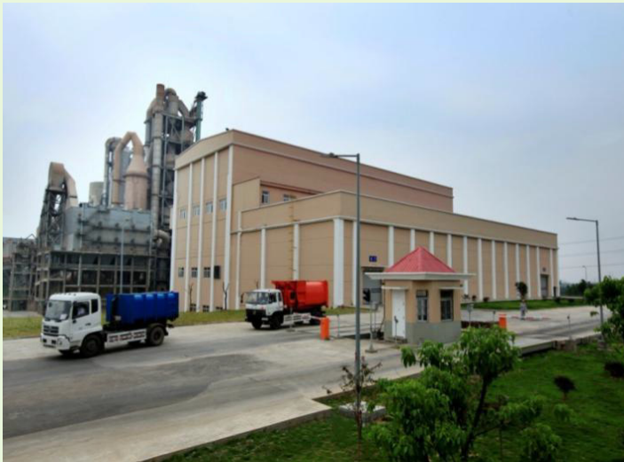
The project of Tongling Conch, Anhui Province was put into operation in April 2010.
