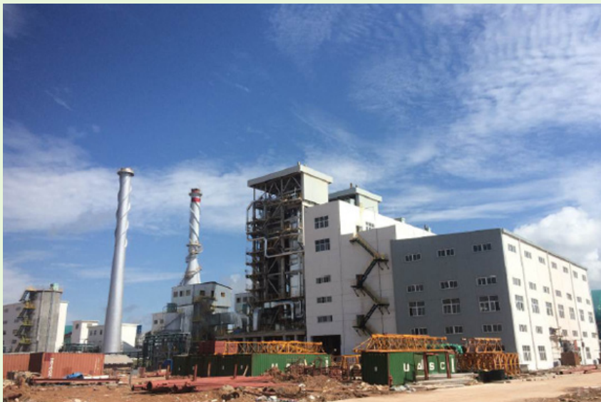
Panorama of Cambodian MCL captive power plant project
