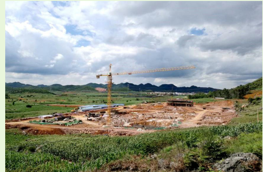
Grate furnace power generation project under construction in Yanshan, Yunnan Province
