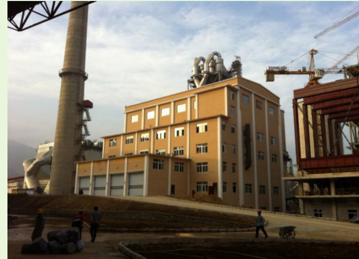
The project of Guiding Conch, Guizhou Province was put into operation in Nov. 2012.
