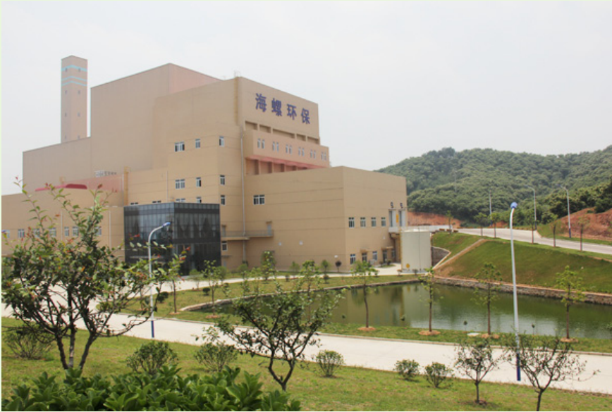
Panorama of grate furnace power generation project in Jinzhai, Anhui Province
