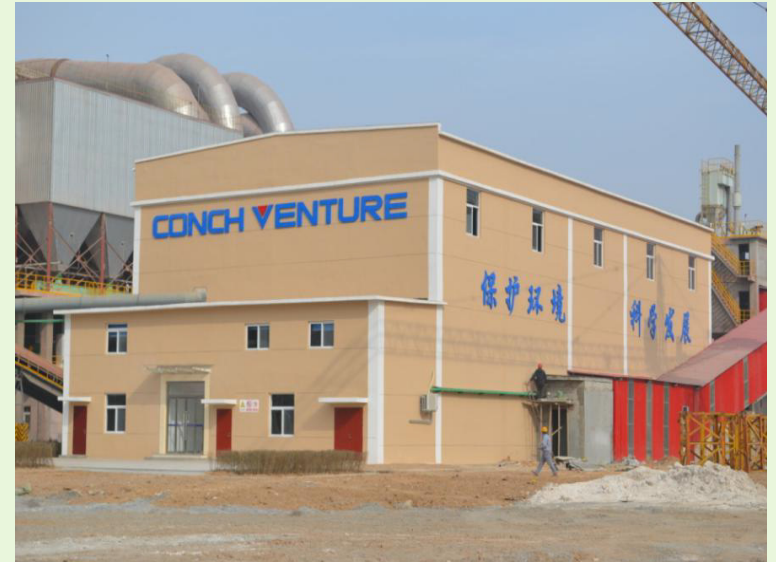
Plant of sewage sludge disposal project under construction in Qian County
